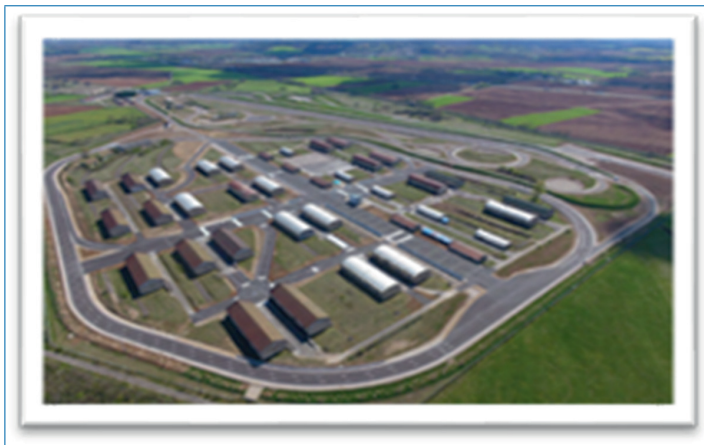
Figure 11.5. Aerial View of the Transpolis site.
