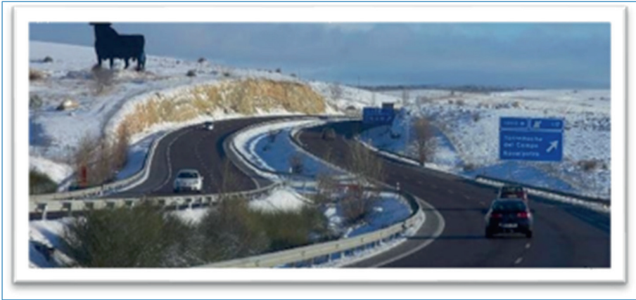
Figure 11.3. Overview of the A2 motorway.
