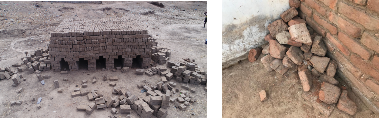
Figure 1.2: The brick clamp: A popular, but wasteful technology.
