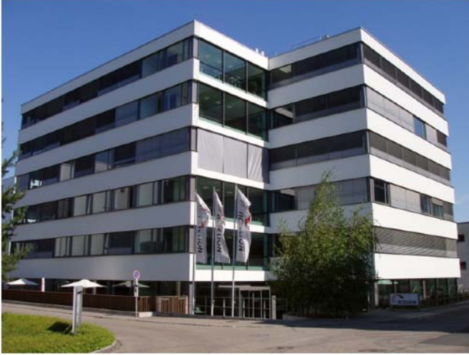
Fig. 1. Building used for the experiments.
