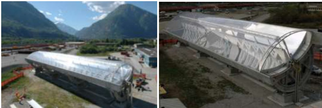
Fig. 4. Photographs of a full-scale 42 m long prototype of the inflated trough concentrator in Biasca, Switzerland. An array of 5 secondary concentrators was placed in the center of the trough [2].
