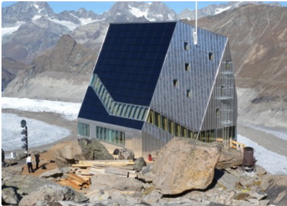
Schmitt, G. 2009. The Monte Rosa shelter produces all of its electricity with photovoltaic elements. [Photograph].
