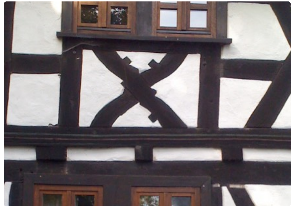
Schmitt, G. 2008. Oak wood, with adobe and straw infill. These local materials help sustain this schoolhouse in Schönberg since 1697. [Photograph].
