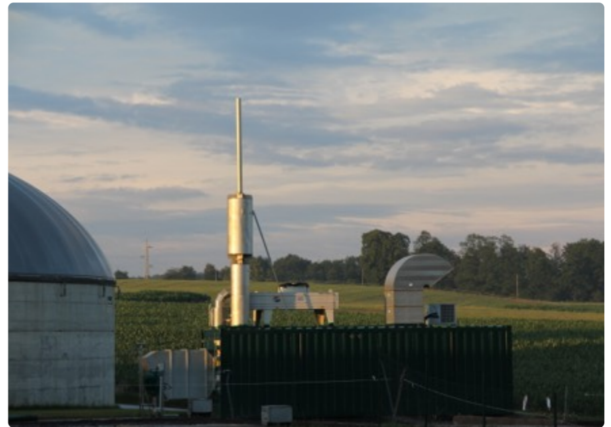
Schmitt, G. 2011. A 265 kW biogas plant supplying electricity for a part of a small town. [Photograph]. Kastanienhof, Wadern, Germany.
