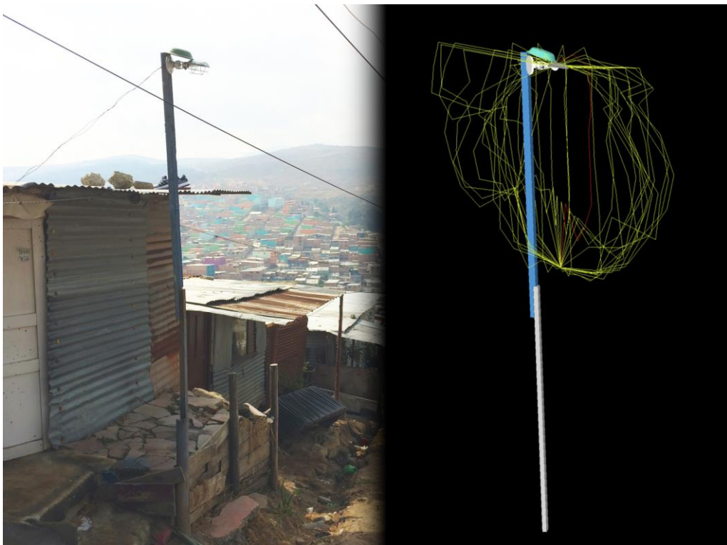
Figure 5. Digitisation Process of Informal Luminaires Including Physical and Photometric Information Source: Kretzer and Walczak, 2020.
