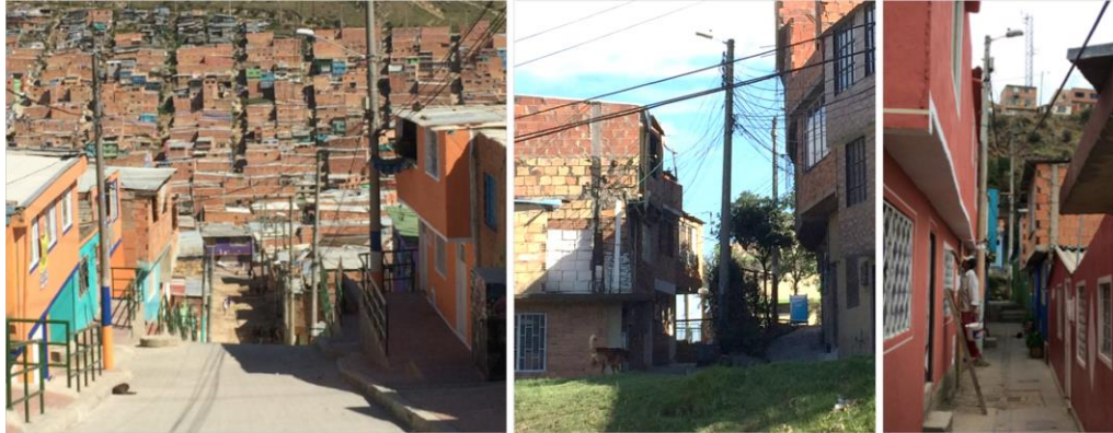
Figure 1. Luminaires of Similar Height Lighting a Nine-Metre-Wide (left-hand side), Less than Six-Metre-Wide (middle) and Less than Three-Metre-Wide (right-hand side) Street
