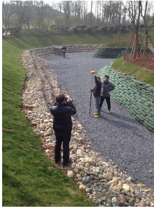
Figure 2: Sponge city in Nanchang, capital city of Jiangxi Province. Local engineers make final height elevation control measurement for a built pond fed by natural infiltration and draining into nearby Jiulong Lake. Credits: Diego Salmeron
