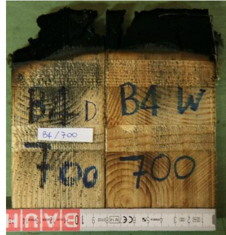
Figure 3: Remaining CS (including the char layer) and residual CS in the length allocated to CS B thermal exposure (measurements at 700 mm)
