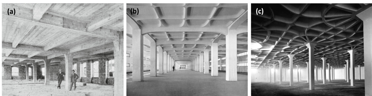
Figure 1. Compilation of historical ribbed floor slabs: (a) Möbelfabrik Reutlinger, Karlsruhe (1899, Photo: CNAM/SIAF), (b) Manifattura Tabacchi, Bologna (1949, [12]), (c) Lanificio Gatti, Roma (1953, [12]).
