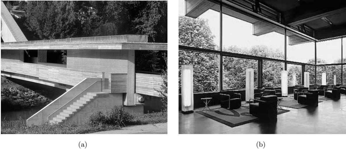
Figure 2.6: 2.6(a): Bridge for pedestrians in Murau, Austria [49] 2.6(b): The “Swiss Re Centre for Global Dialogue” with post-tensioned timber beams [50]
