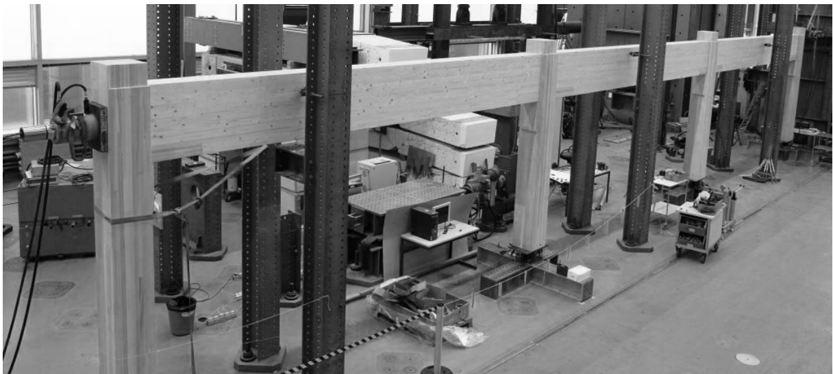
Figure 5.2: Three-bay post-tensioned timber frame for pushover tests on the strong floor at the ETH Zurich
