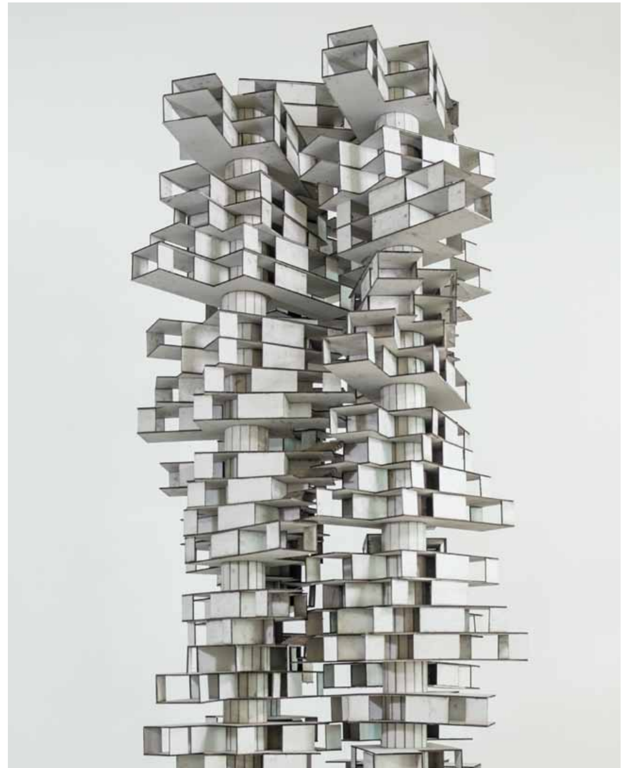
Tower 2 In the second tower the void decks are introduced. Every sixth floor is left empty, articulating clusters of residential units. These clusters act as Vierendeel trusses, leaving the void decks free of structure. The apartments rotate freely around their centre, creating different views and trying to connect to the next void deck cluster.
