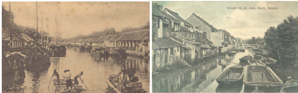
Figure 4.4.9: Left – 1907 view of the Kali Besar (Ciliwung River) near the sea. Right - 1912 view along one of the canals near the Java Bank, illustrating access-ways and the canal's profile. Source: Merrilees [147].
