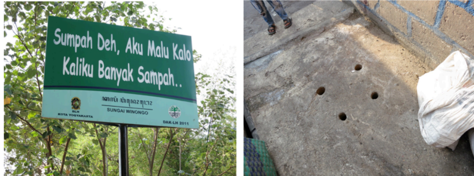
Figure 3.4.7: Left, a sign in a park along the Winongo River, Yogyakarta, reads 'I swear, I'll be embarrassed should my river be filled with trash'. Right, Biopori have been drilled through hard surfaces in a riverside neighbourhood to increase permeability. Author's fieldwork, 2012.
