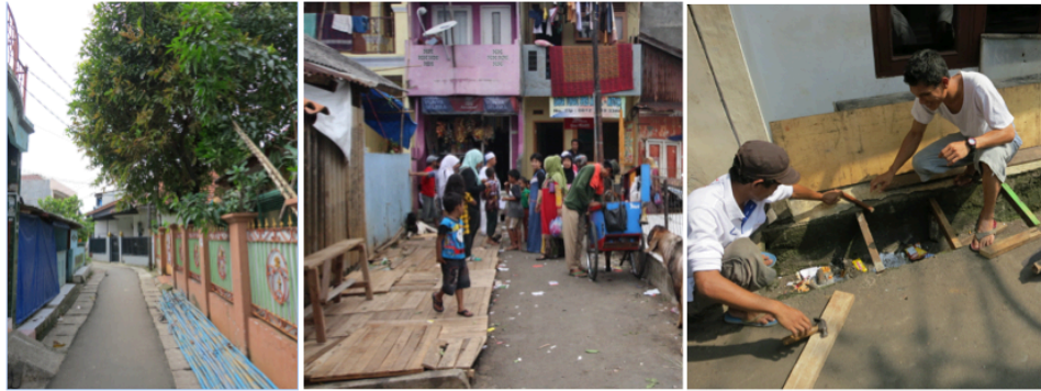
Figure 5.2.16: In areas where space is limited drains are often covered to increase street capacity. While concrete drain covers are most commonly used (Left), less durable materials such as timber may also be used to provide coverage to increase space (Centre and Right).
