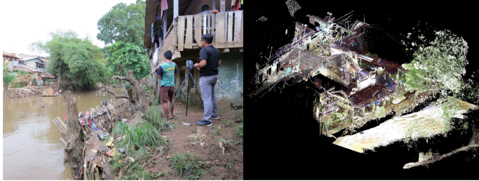
Figure 2.2.6: Left - Capturing the Bukit Duri site model using the terrestrial laser scanner with the help of the NGO collaborator; Right - Sample of the Bukit Duri site model. Source: [193]
