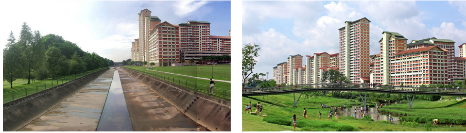
Figure 1.3.5: Bishan Park, Singapore (Left) Before the removal of the concrete drainage channel (Right) After the channel was naturalised. Source: Ramboll Studio Dreiseitl.
