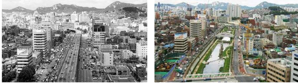
Figure 1.3.6: Re-daylighting the Cheongyecheong Stream in Seoul, South Korea (Left) The highway over the culverted Cheongyecheong, before the re-daylighting; (Right) After the re-daylighting. Source: [233]
