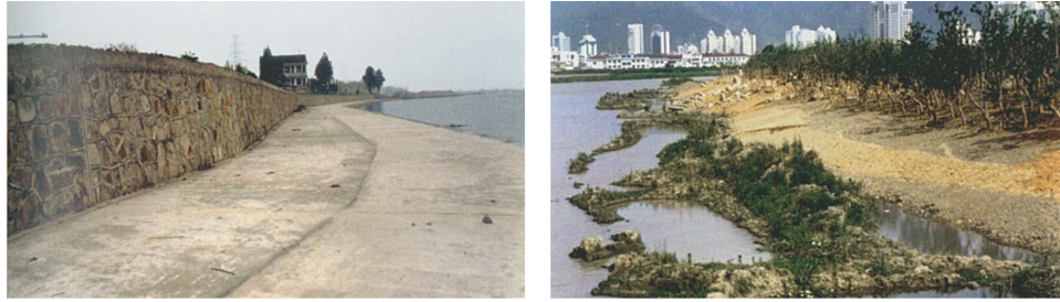
Figure 1.3.4: Yongying River Park in Taizhou, China, (Left) before the removal of a concrete embankment (Right) regrading process required to restore riparian edges. Source: Water Urbanisms East [57].
