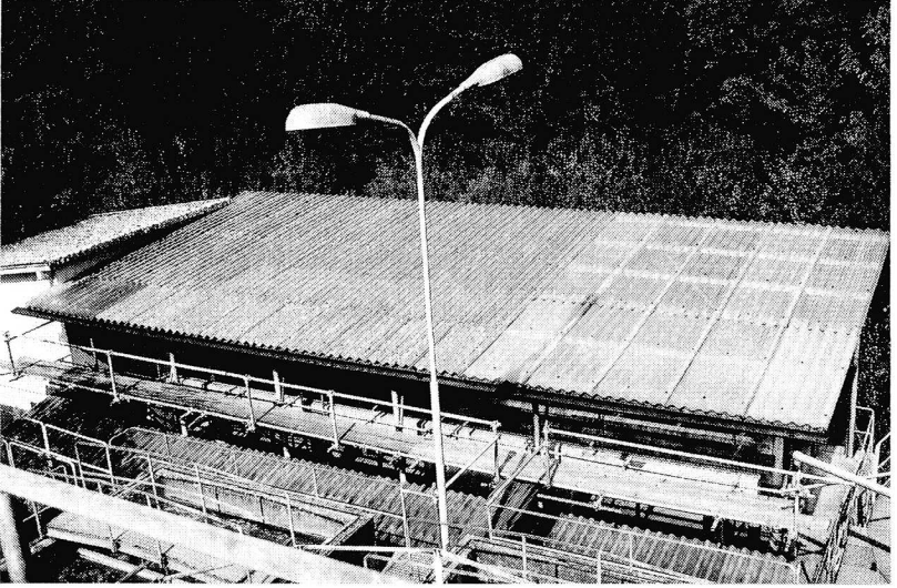
Figure 4.3 Polyester roof in Tüffenwies.
