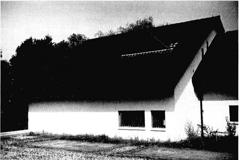
Figure 4.4 Clay tile roof at Werdinsel.
