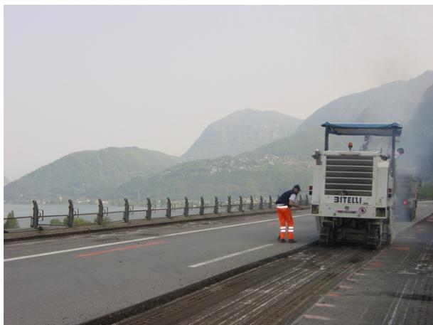
Figure 45: Pavement removal with milling machine.
