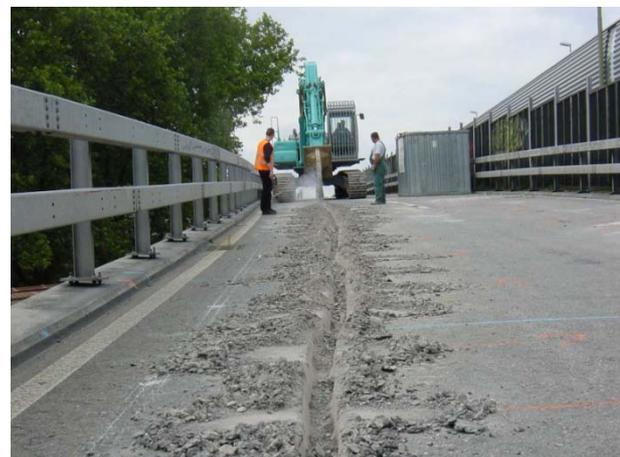
Figure 46: Pavement opening with excavator.
