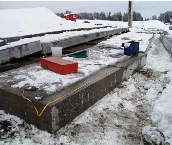
Figure 43: Sawed bridge deck.
