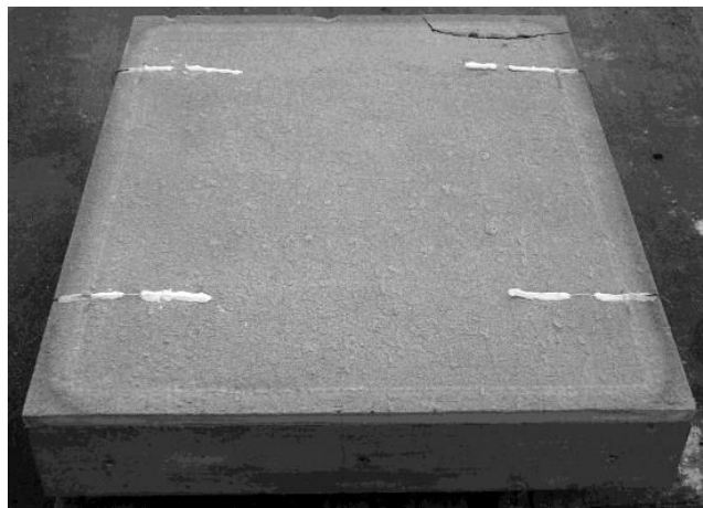
Fig. 5.13 HPC slab with 20 mm of protective mortar after 120 minutes of ISO fire exposure.
