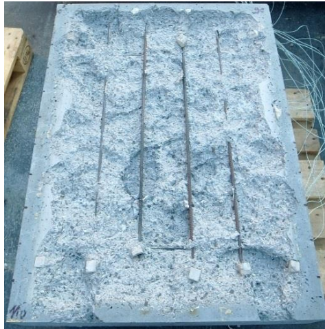
Fig. 1.1 Explosive spalling of a concrete slab (Lu & Fontana 2015).
