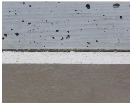
Fig. 5.31 HPC slab protected by insulation plate.
