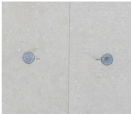
Fig. 5.46 The joint of plates on the protected HPC slab.
