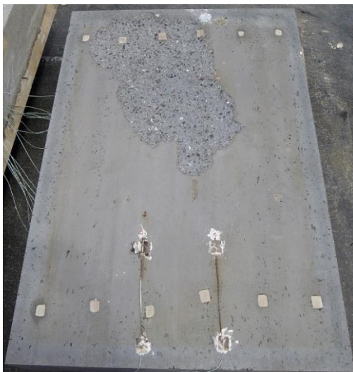
Fig. 4.5 Spalled HPC slab after 14 minutes of fire exposure.
