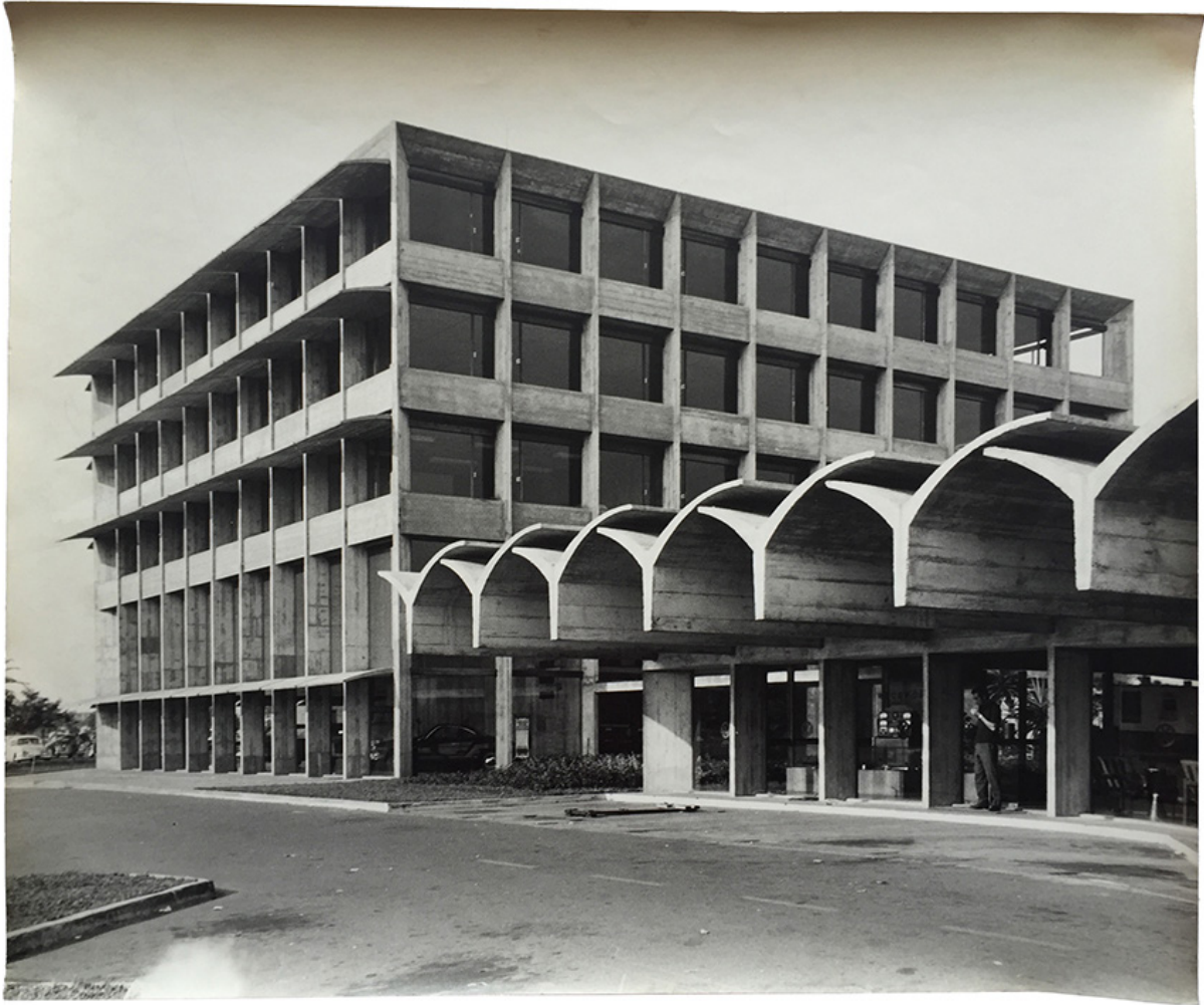
Fig. 1.37 Disbrave building. View of the Office Block. João Filgueiras Lima, 1965. Photograph by Marcel Gautherot. Arquivo João Filgueiras Lima, Salvador
