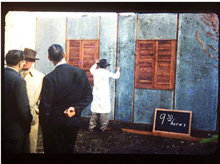
Fig. 2.50 The Uni-Seco system. Assembly of prefabricated houses designed by the architect Eduardo Kneese de Mello (1954) in Jaboticabal, São Paulo state. During the inauguration event, a notice plate was hung at the end of each stage of the assembly process showing the respective time spent on construction. Roberto Montenegro, "A pré-fabricação na trajetória de Eduardo Kneese de Mello" (PhD diss., Universidade de São Paulo, 2012), 103. Arquivo FEBASP
