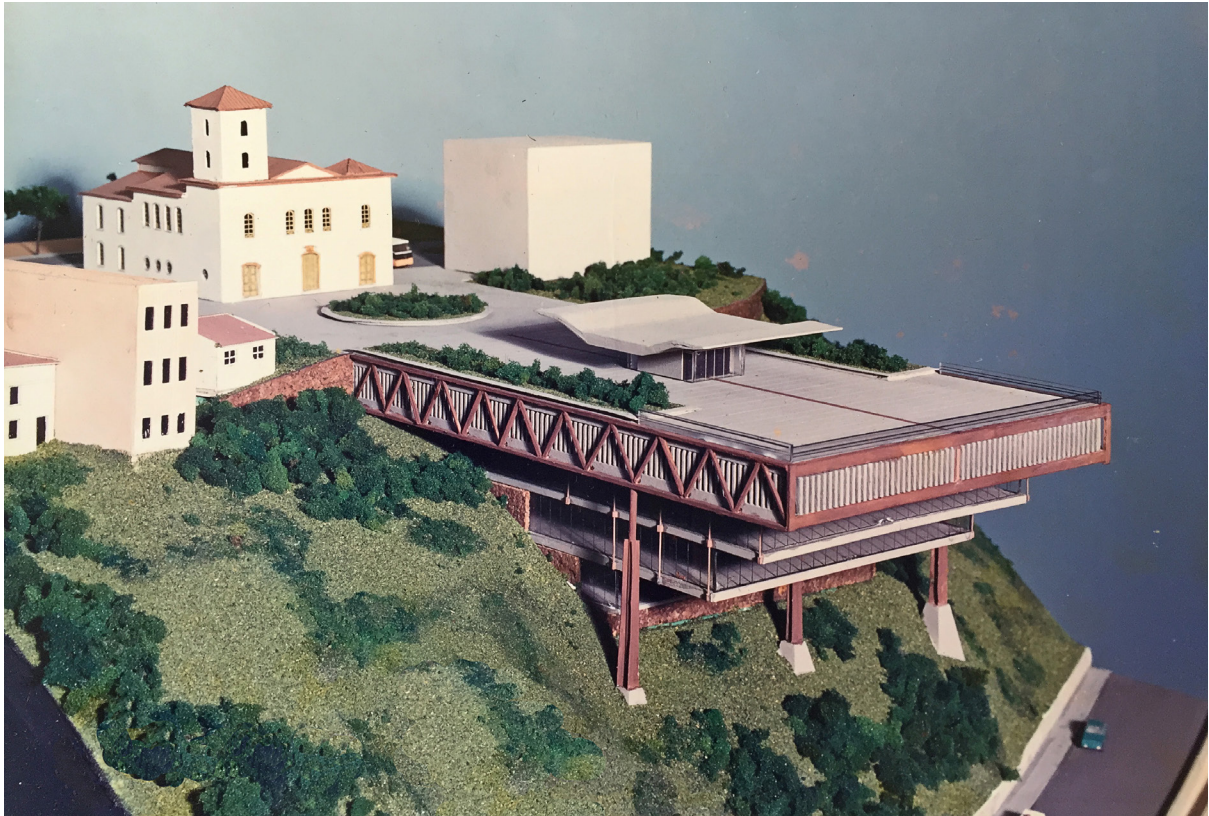
Fig. 2.120 Lelé's proposition for the Largo dos Afritos square in Salvador, 1988. Above: Scale model showing the inverted staggered structure built into the hill, with a marquee at the center. Below: Longitudinal section. Arquivo João F. Lima, Salvador
