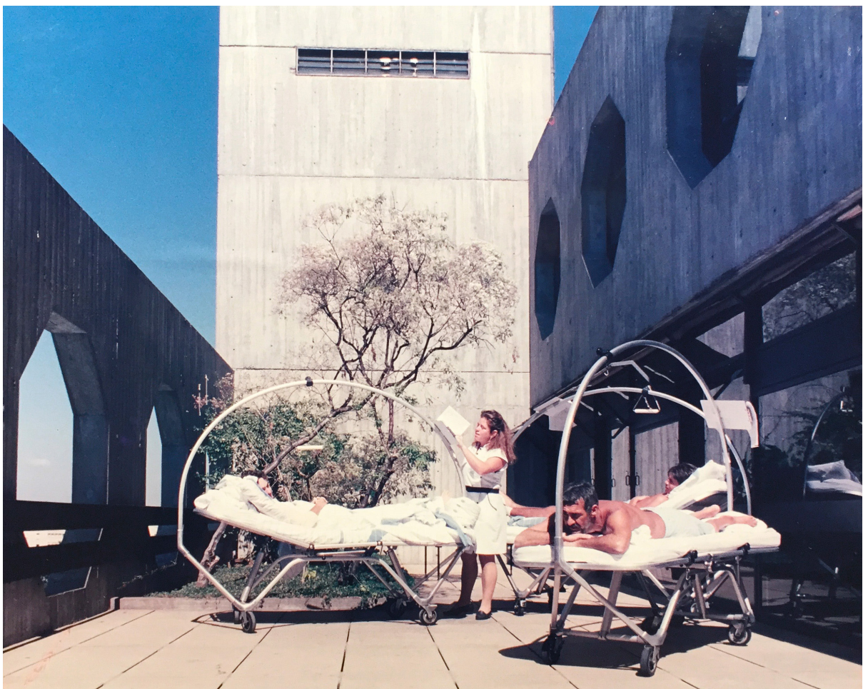
Fig. 1.47 Solarium and the cama-maca (mobile bed). Sarah rehabilitation hospital in Brasília. João Filgueiras Lima, 1976-80. Arquivo João Filgueiras Lima, Salvador
