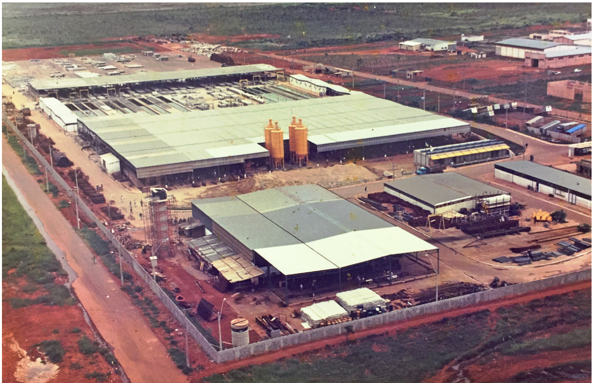
Fig. 3.50 Aerial view of the Argamassa Armada Factory in Brasília (Ceilândia satellite city) displaying the expansion of the facilities. Arquivo Aires Carvalho, Brasília
