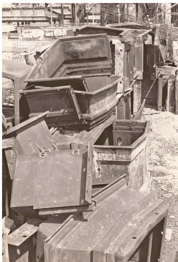
Fig. 3.11 View of the drainage stairways' metallic molds ( módulo drenante ) at the production patio of RENURB. Salvador, 1981. Arquivo Kristian Schiel, Brasília
