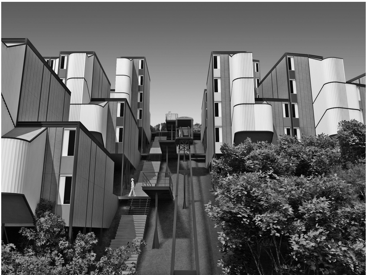
Fig. i.v View of the funicular railway of the housing complex at the district of Pernambuco, Salvador. Project by Lelé, 2011. Arquivo Instituto Brasileiro de Tecnologia do Habitat (IBTH), Salvador
