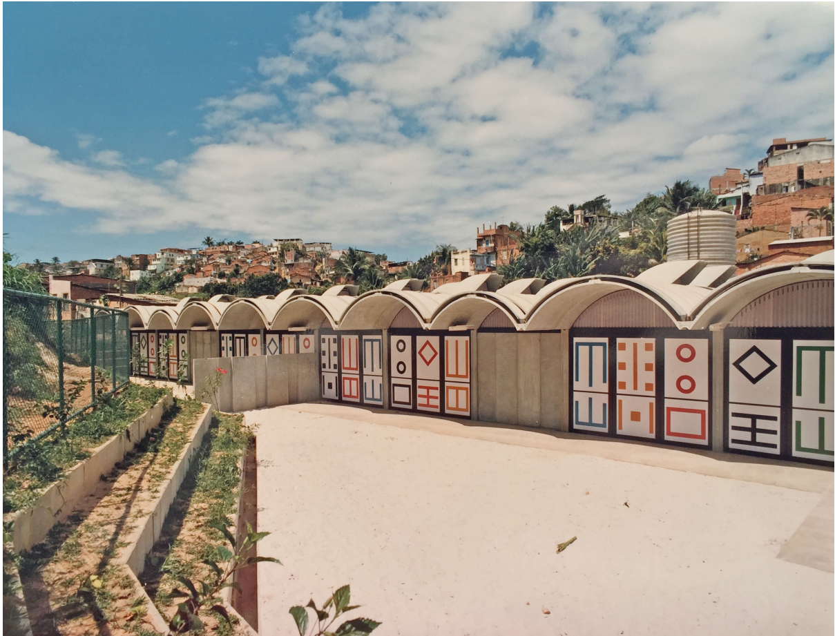
Fig. 2.83 Vaulted-roof kindergarten in the district of Bom Juá, Salvador. Design by Lelé, 1987. Photograph by Celso Brando. Integrated arts by Athos Bulcão. Arquivo João Filgueiras Lima, Salvador
