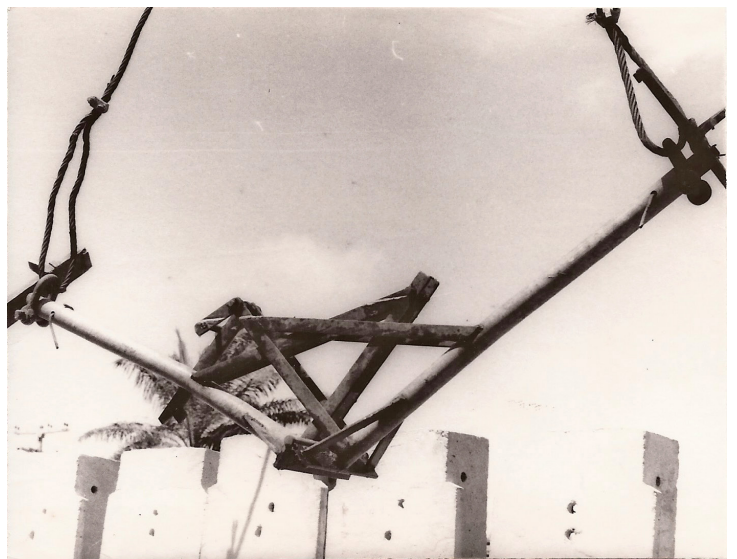
Fig. 3.22 Lifting device developed at RENURB. A metallic articulated bar hung by steel cables. Salvador, 1980. Arquivo Kristian Schiel, Brasília
