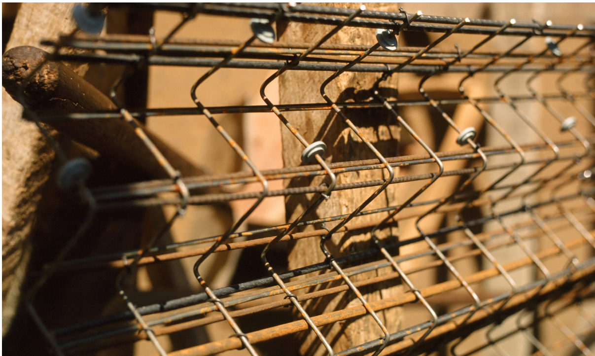
Fig. 1.62 Plastic spacer. Top left: Lelé's sketches detailing the object dimensions and production estimation. Arquivo Kristian Schiel, Brasília | Top right: samples of the spacer from the CTRS factory in Salvador. Photograph by the author | Bottom: Application of the spacer in the welded steel mesh of a precast argamassa armada element. Arquivo Kristian Schiel, Brasília
