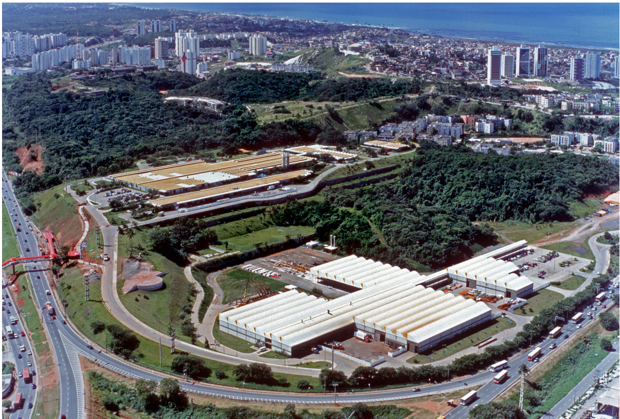
Fig. 3.67 Aerial view of the hospital and the factory in Salvador. The expansion area of the CTRS (dedicated to the post-graduation courses) remains undeveloped (on the right). Arquivo João Filgueiras Lima, Salvador
