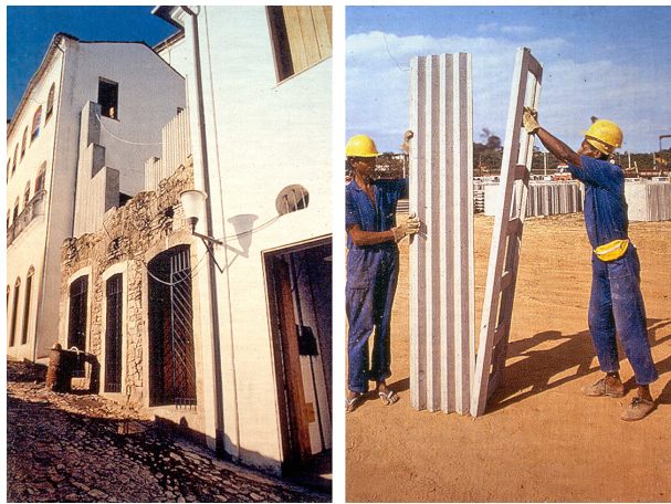
Fig. 2.77 Intervention at Ladeira da Misericórdia in Salvador (in collaboration with Lina Bo Bardi). FAEC, 1987-88. Arquivo João Filgueiras Lima, Salvador
