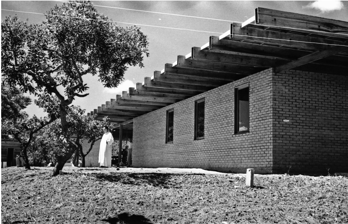
Fig. 1.21 Friar Mateus' residence and chapel at the University of Brasília (UnB). João Filgueiras Lima, Brasília, 1962. Arquivo Central da Universidade de Brasília
