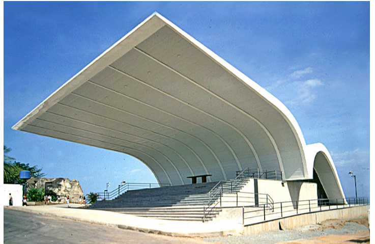
Fig. 2.126 São José de Ribamar Chapel (1997). Both marquee and bell tower were produced in Salvador and delivered disassembled to São Luís region (1573 km from Salvador) in the north-east of Brazil. Arquivo João Filgueiras Lima, Salvador
