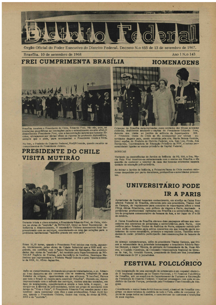
Fig. 3.3 President Frei visited a self-build cooperative (mutirão) in Brasília, where low-income houses were produced close to the capital's industrial sector. Arquivo TCDF. Available at : http://www.tc.df.gov.br/SINJ/Diario/ Accessed on September 19, 2017
