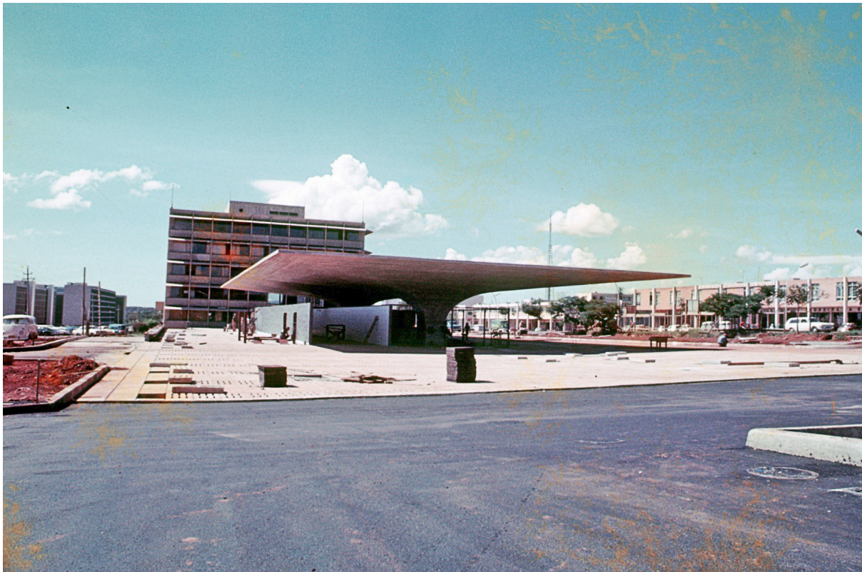
Fig. 2.123 Disbrave gas station under construction. The imposing marquee is part of the building complex expansion project designed by Lelé in 1975, in Brasília. Arquivo João Filgueiras Lima
