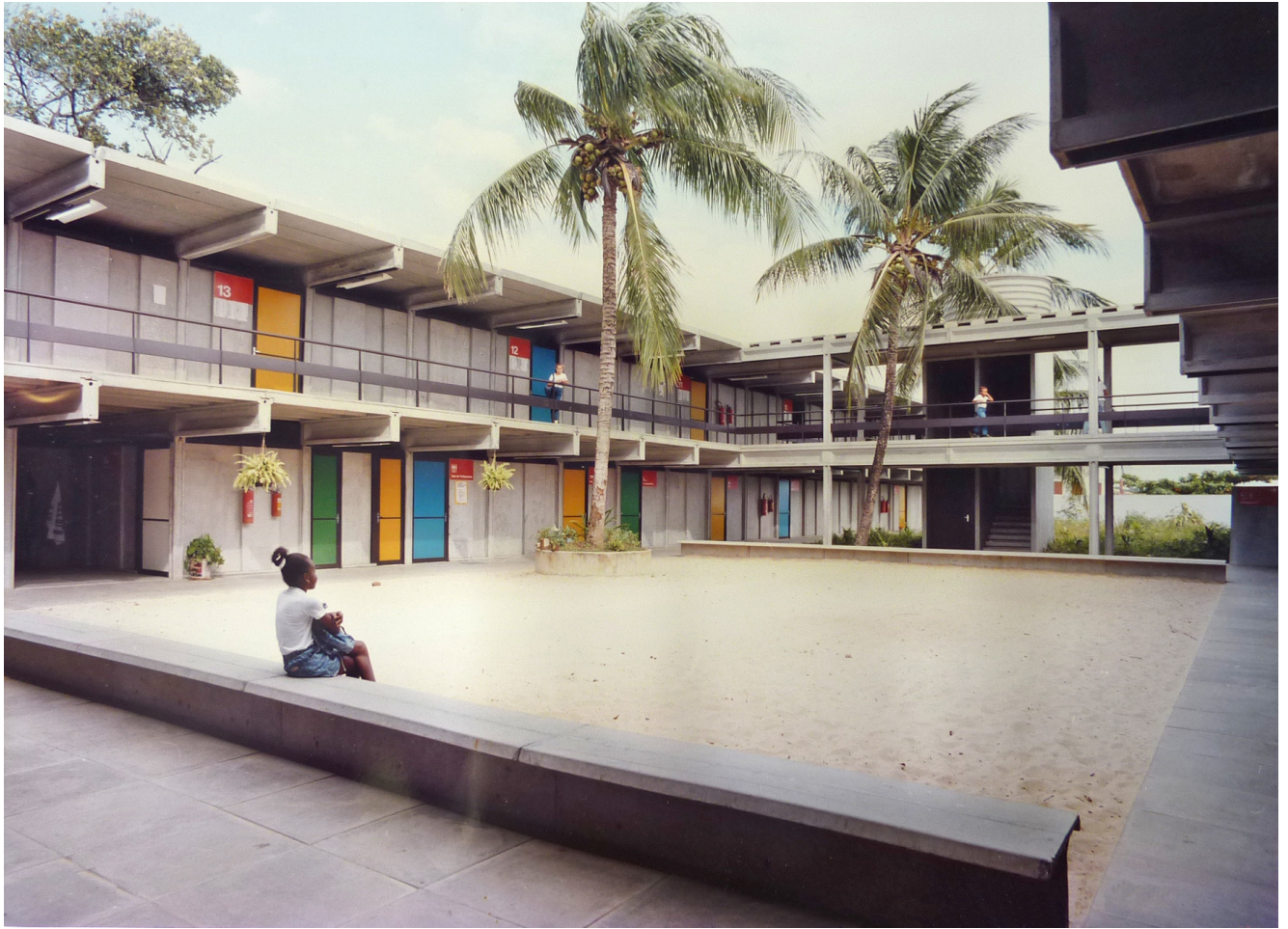
Fig. 2.89 Two-story prefabricated school produced and assembled by FAEC in Salvador (1986-88), Beirú district. Design by Lelé, photograph by Celso Brando. Arquivo João Filgueiras Lima, Salvador
