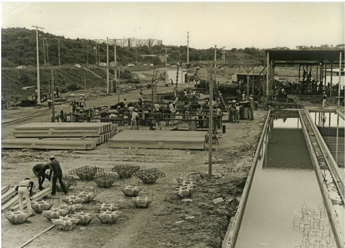
Fig. 3.53 The City Factory (FAEC) in Salvador. Above: aerial view of the plant's facilities in the district Caminho das Árvores . Below: Faec's production area showing the curing tanks and some precast elements, such as the gutter-beam and the star-shaped foundation. Arquivo Fundação Gregório de Mattos, Salvador
