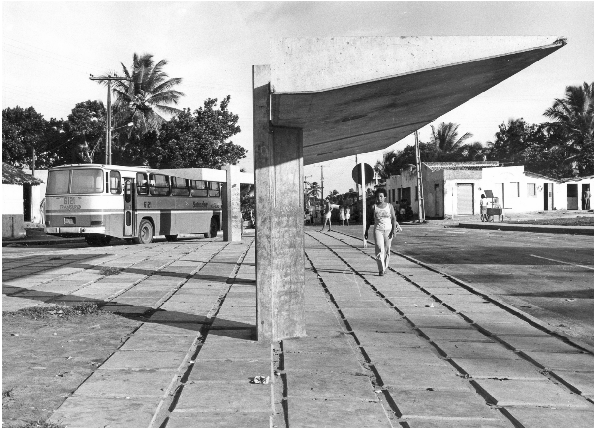
Fig. 2.16 RENURB bus shelter model for Salvador, Bahia. Precast reinforced concrete. Design by Lelé, 1979. Arquivo João Filgueiras Lima, Salvador
