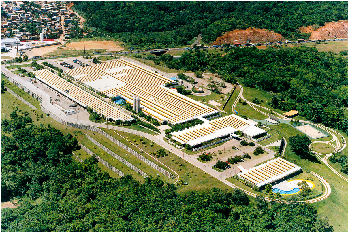
Fig. 2.98 Aerial view of the Hospital Sarah Kubitschek in Salvador, a project which began in 1987. Design by Lelé. Arquivo Instituto Brasileiro de Tecnologia do Habitat (IBTH), Salvador
