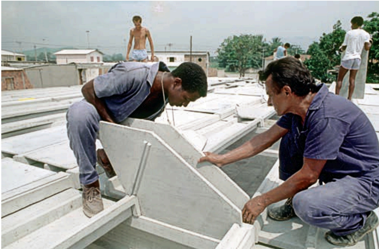
Fig. 2.109 Assembly process of a shed in Rio de Janeiro. Lelé modified the element before it entered mass production at the School Factory. An acrylic shutter was designed to protect the roof opening from direct sunlight. Marina Mange Grinover, PhD diss., (Universidade de São Paulo, 2015), 346
