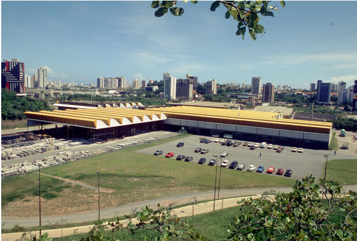
Fig. 3.71 External view of the CTRS's argamassa armada workshop showing the small storage area for the precast elements. Arquivo João Filgueiras Lima, Salvador
