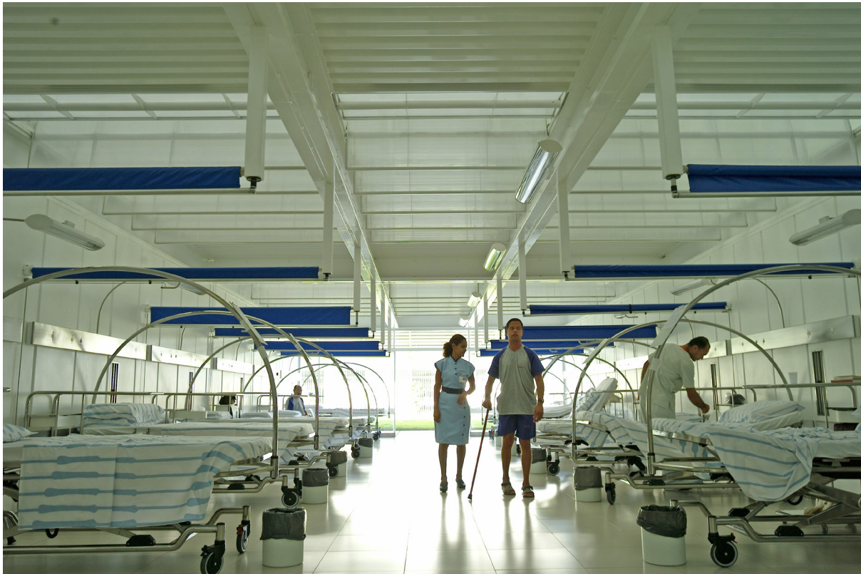
Fig. 2.113 Medical wards of the Sarah Rehabilitation Hospital in Rio de Janeiro, Lelé, 2009. When the motorized air dumper ceiling is opened (as in the picture above) it means that there is an exchange of air between the airflow from the rooftop and the space below. Photograph by Celso Brando. Arquivo João Filgueiras Lima
