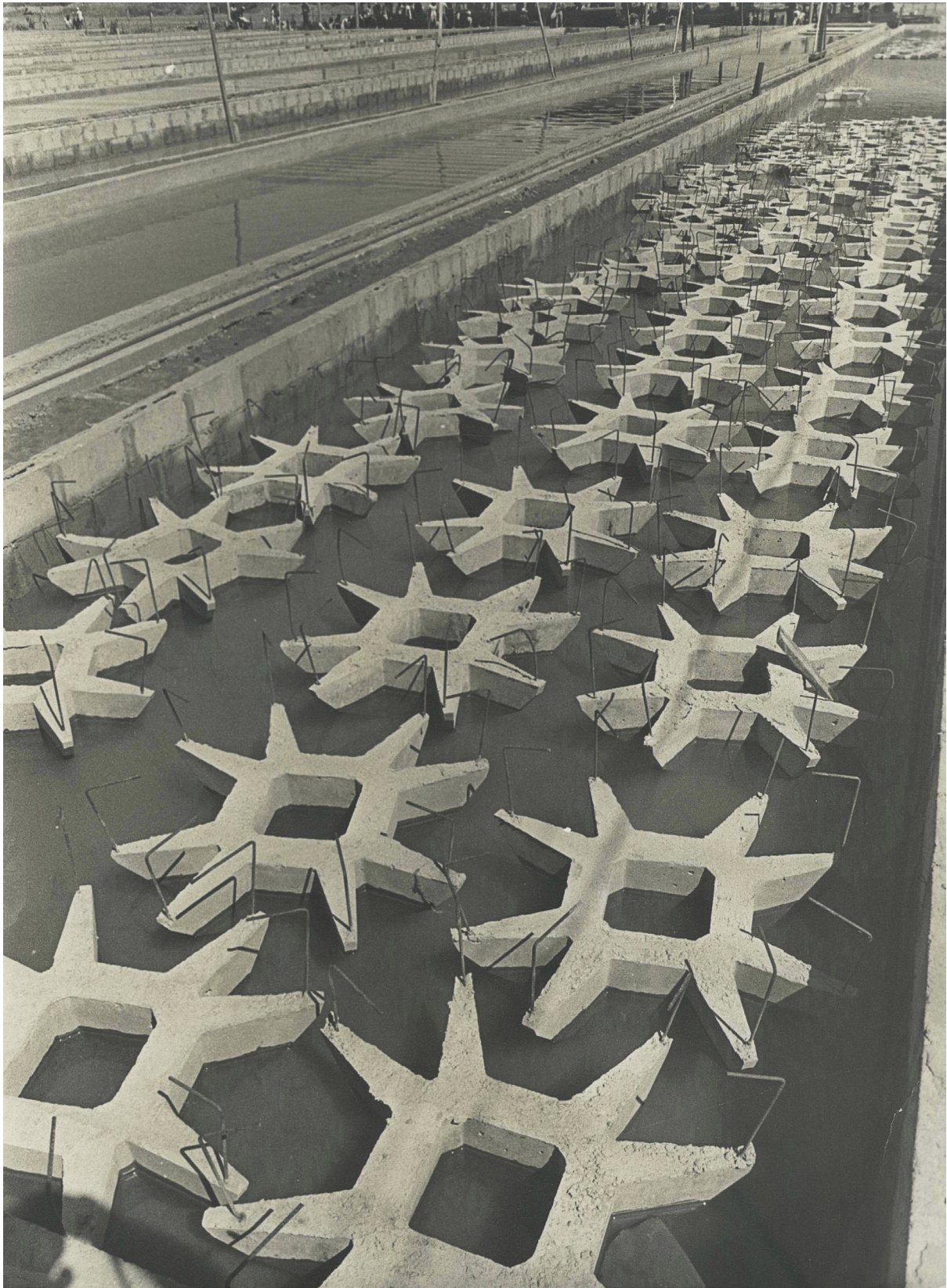
Fig. 2.87 A cure tank with a series of star-shaped foundation elements made of argamassa armada . A major feature of the primary schools. FAEC factory, Salvador. Design by Lelé, 1986. Arquivo Fundação Gregório de Mattos, Salvador, 2016
