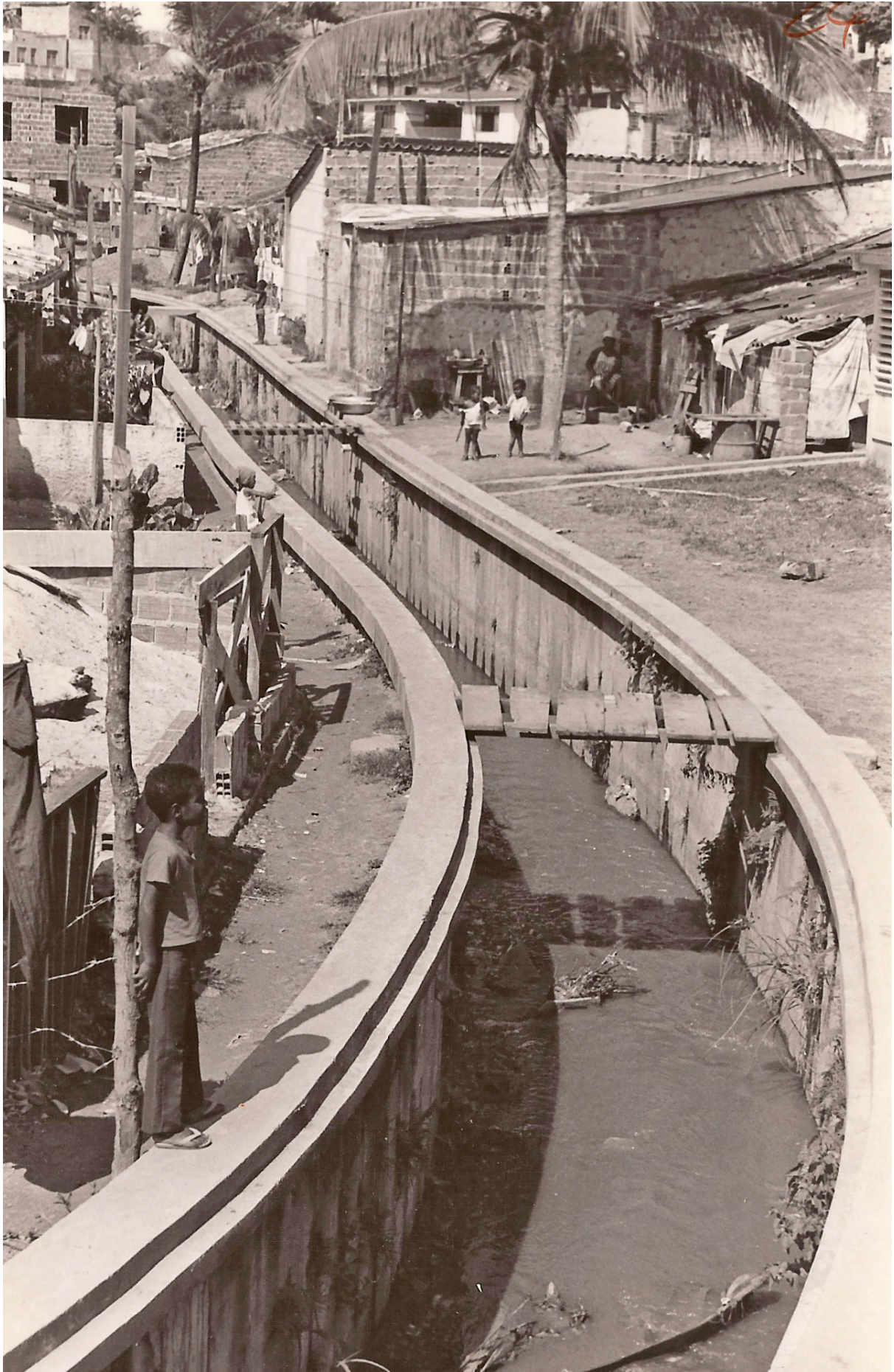
Fig. 2.39 Accomplished channel in a poor neighborhood of Salvador. (1980) Arquivo Kristian Schiel, Brasília
