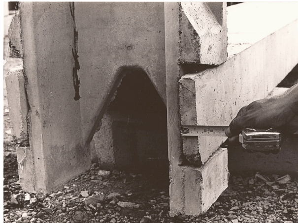
Fig. 2.38 Sanitation channel precast element in argamassa armada , Salvador, 1980. Connection between a wall and bottom element through the drawer groove (final solution). Component thickness: 3 cm. Arquivo Kristian Schiel, Brasília
