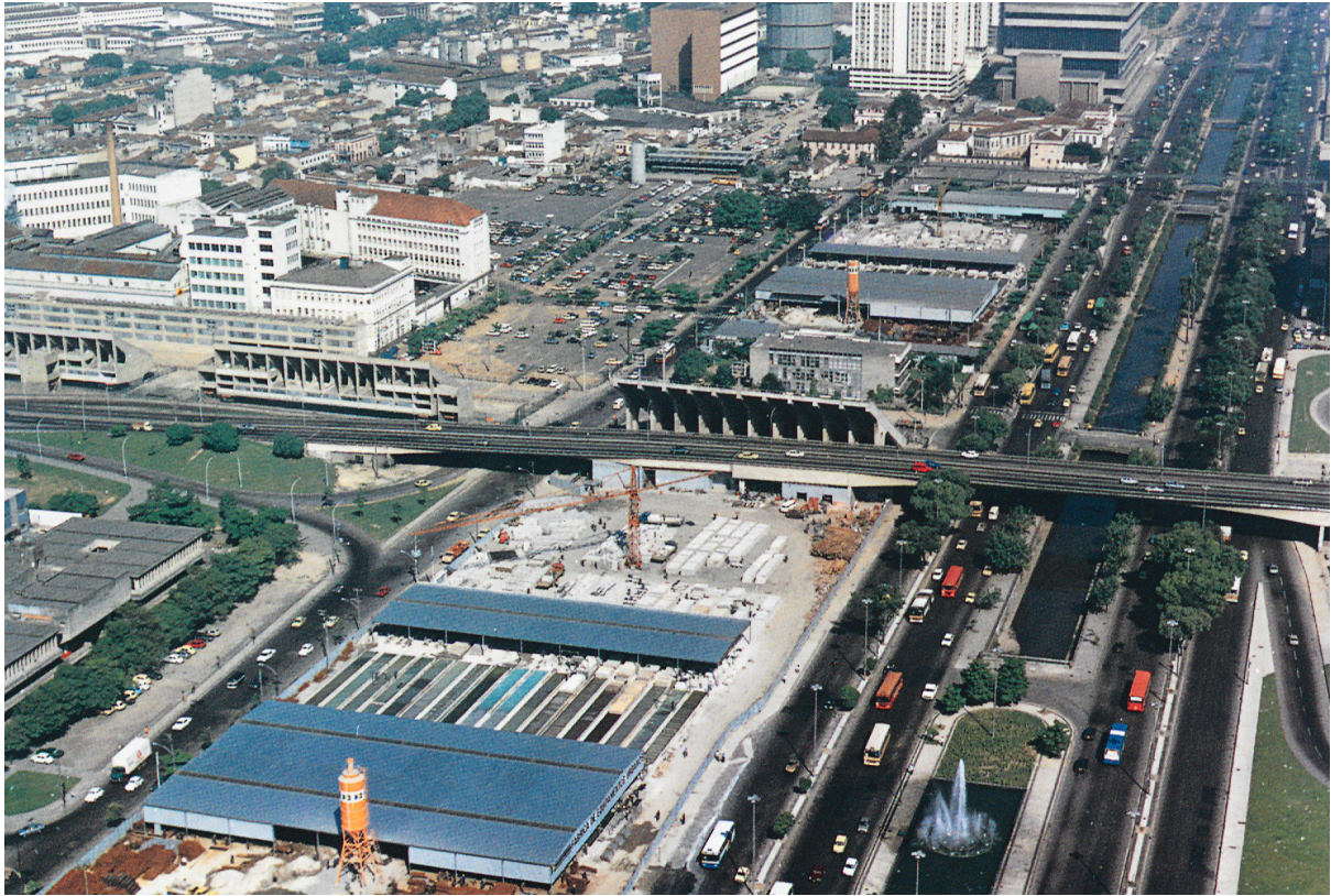
Fig. 3.43 The School Factory after the expansion of its facilities in the city center. Rio de Janeiro, 1985. Giancarlo Latorraca. João Filgueiras Lima, Lelé . Edited by Marcelo Carvalho Ferraz. Lisboa, São Paulo: Editorial Blau, Instituto Lina Bo e P.M. Bardi, 2000, p. 148
