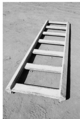
Fig. 1.9 Prefabricated pleated walls (buttress) in argamassa armada, Salvador, 1988. Giancarlo Latorraca, João Filgueiras Lima, Lelé (Lisboa: Blau, 2000), p. 168
