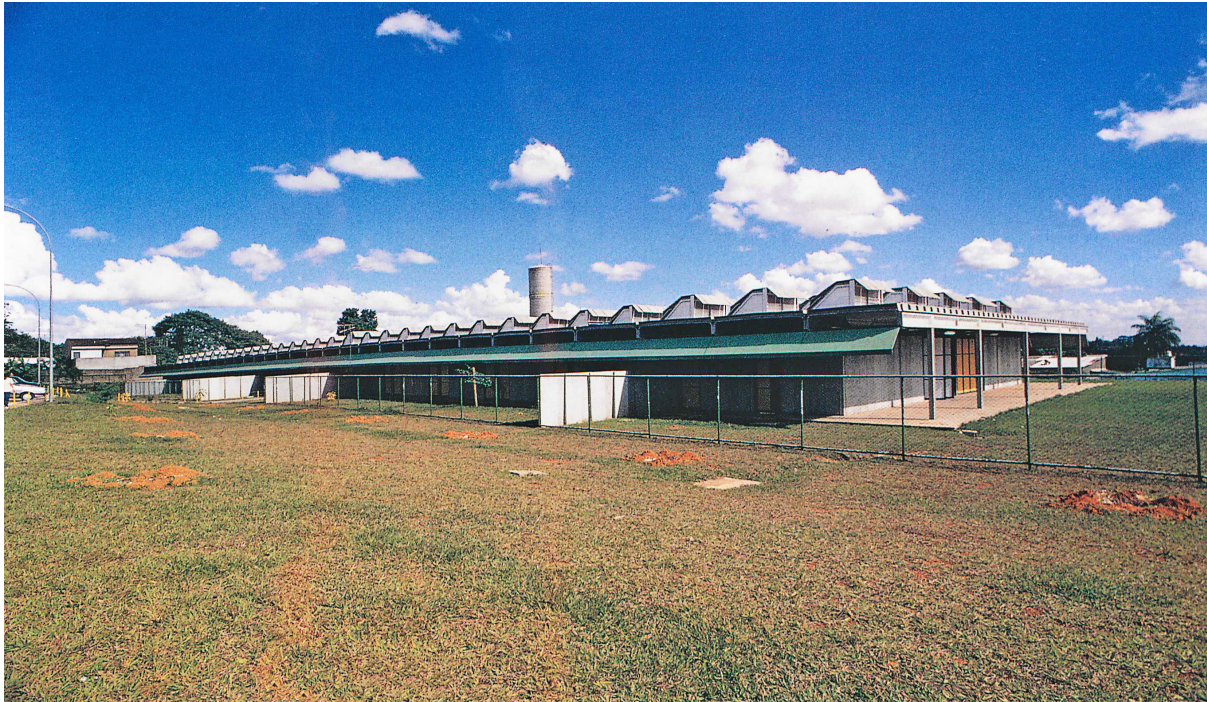
Fig. 2.102 Psychiatric Hospital of Taguatinga. Main façade showing the sequence of isolated roof sheds. Architect João Filgueiras Lima. Taguatinga, Distrito Federal, 1987-88. Giancarlo Latorraca, ed. Marcelo Ferraz, João Filgueiras Lima, Lelé (São Paulo: Instituto Lina Bo e P.M. Bardi; Lisboa: Editorial Blau, 2000), p. 165
