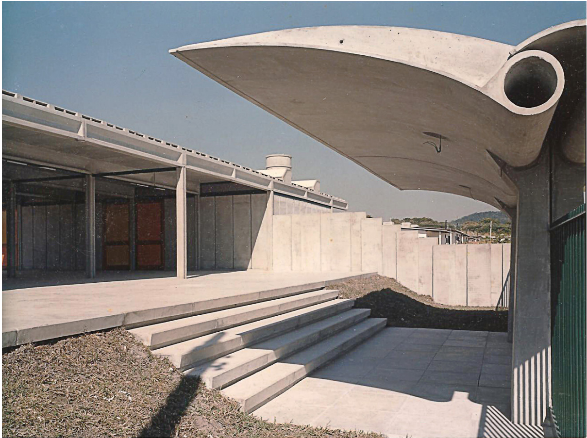
Fig. 2.23 Precast bus shelter in argamassa armada developed by Lelé in Rio de Janeiro (1985) as part of the governmental program Fábrica de Escolas (School Factory). Photograph by Celso Brando. Arquivo Zeca Franco, Rio de Janeiro
