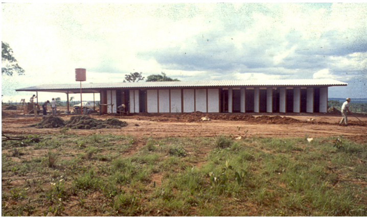
Fig. 2.53 Prefabricated wooden school for 30 students. Lelé, Abadiânia, 1983. Arquivo João Filgueiras Lima, Salvador
