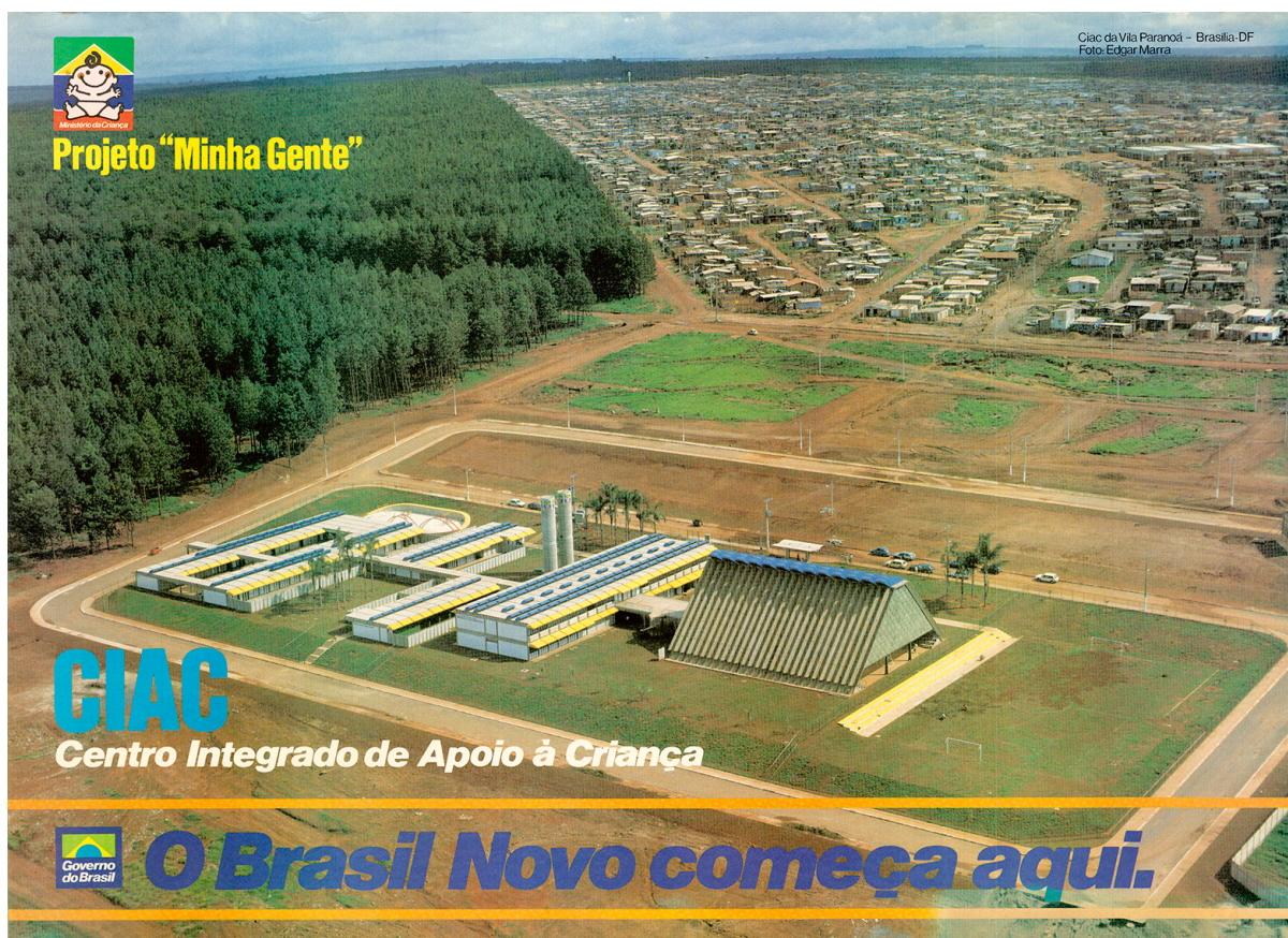
Fig. 2.92 Official poster of the CIAC project ( Minha Gente ). Aerial view of the first prototype assembled in the outskirts of Brasília. Design by Lelé and his team (1991), photograph by Edgar Marra. Arquivo Aires Carvalho, Brasília
