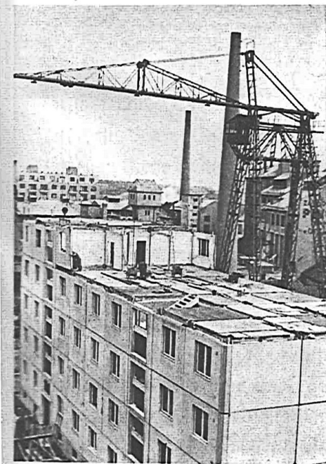
Fig. 1.23 BA System prototype (identical to early paneláks ). V. Karfík, J. Harvančík, K. Šafránek, and team. Bratislava, 1955. Kimberly Elman Zarecor, Manufacturing a Socialist Modernity (Pittsburgh: University of Pittsburgh Press, 2011), p. 275
