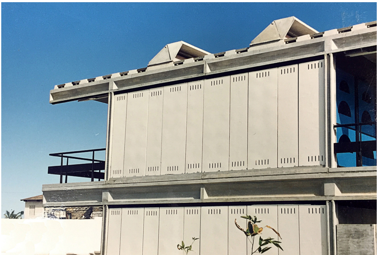
Fig. 2.108 Shed development over Lelé's practice. Shed version of the ground-floor school, 1984 (on the left) and its redesign for the two-story prefabricated school, 1986 (below). Arquivo Aires Carvalho, Brasília
