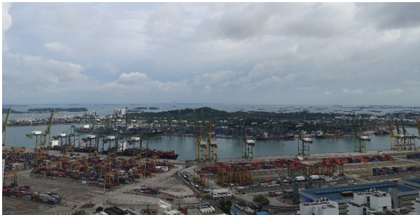
view of Brani Island from the top of Pinnacle at Duxton
