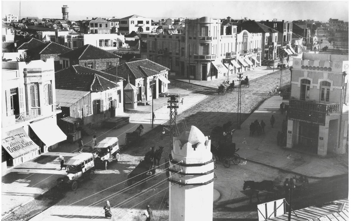
fig. 2 Tel Aviv, Allenby Road, corner Nachlath Binjamin, 1920s.
