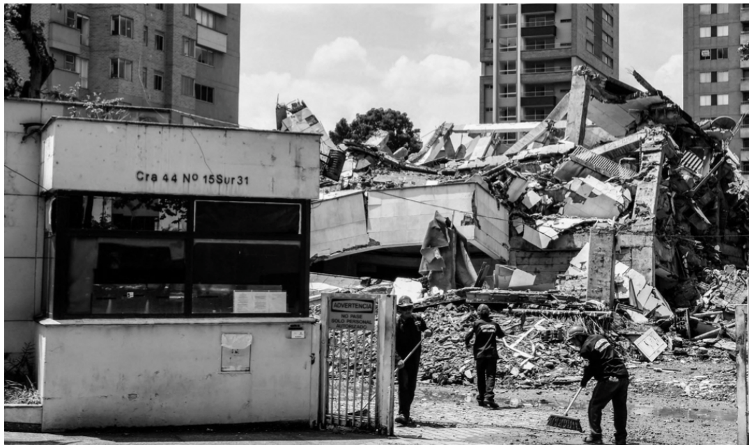
Demolition of Narcos Apartment
