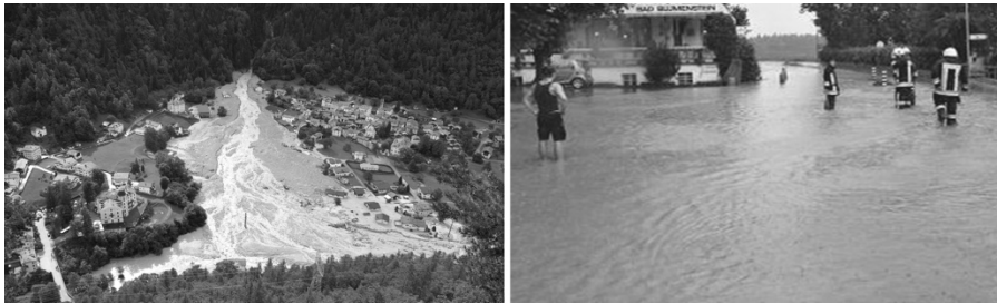
Fig. 3: Left: The alpine village Bondo in Canton Grisons after the debris flow of summer 2017. Large parts of the village were covered and infrastructure destroyed by this natural hazard. Right: Flooding of the Guerbe River in summer of 1990. Due to unexpected heavy rainfall the existing concrete check dams could not withstand the debris flows nor hold large amounts of water.
