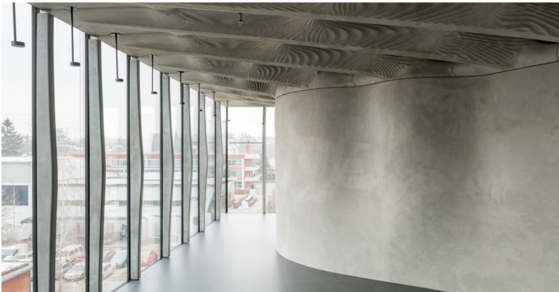
Figure 1.1: Interior of the dfab-house, EMPA, Zürich. Left: Mullions produced by Smart Dynamic Casting. Top: Smart Slab. Right: Multi-curvature Mesh Mould wall (Photo: Roman Keller)
