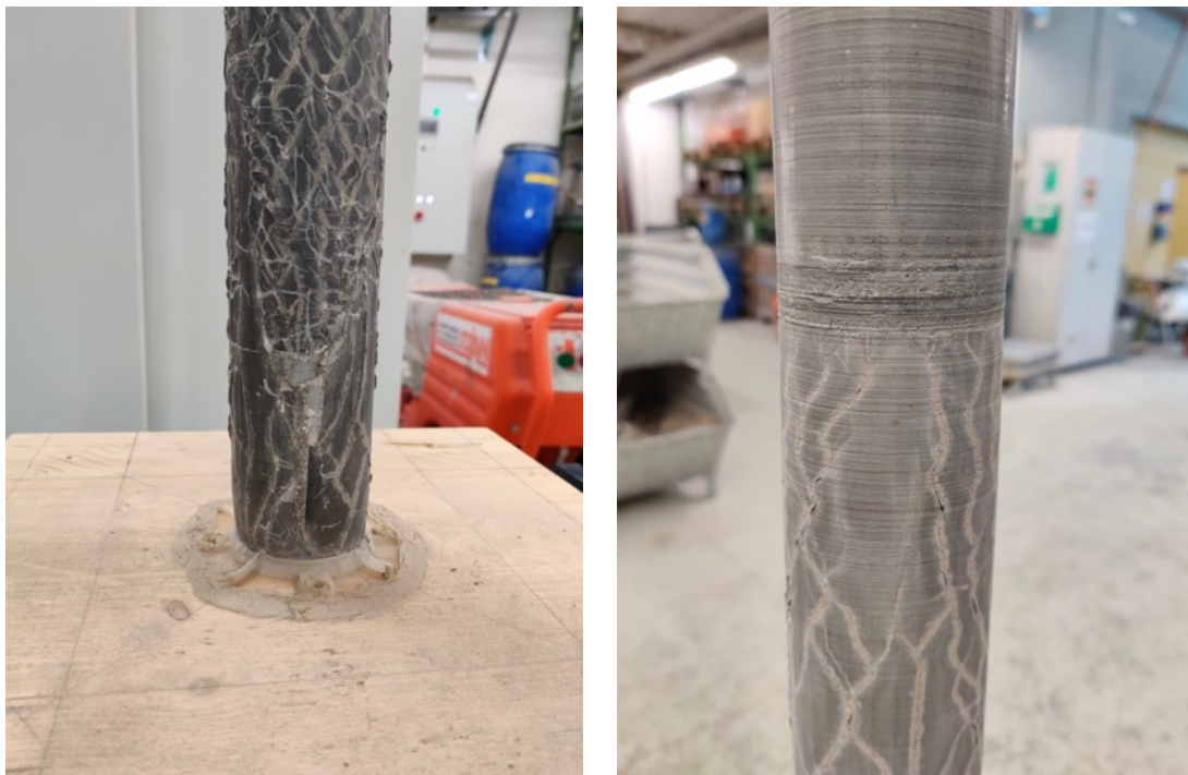
Figure 5.27: Surface details of the lower half of the tube after removing the plastic formwork. Left: Detail of the bottom of the element. Right: Detail of the middle of the element at the level of the cold welding of the two formwork halves.
