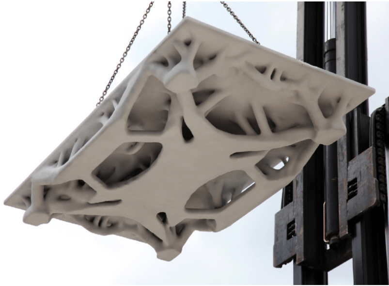
Figure 1.2: Topologically optimised ceiling element. (Photo: dbt, ETH Zürich)
