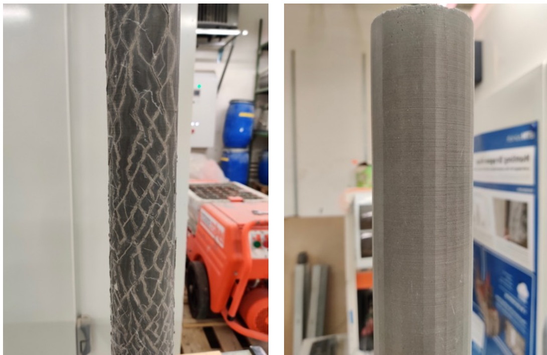
Figure 5.26: Surface details of the tube element after removing the plastic formwork. Left: Detail of the lower half. Right: Detail of the upper half.
