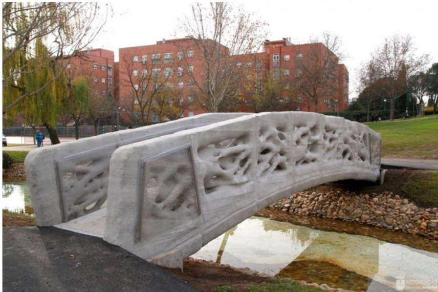
Figure 2.12: Powder-bed 3D printed pedestrian bridge in Castilla-La Mancha urban Park in Alcobendas, Madrid. (Photo: IAAC)
