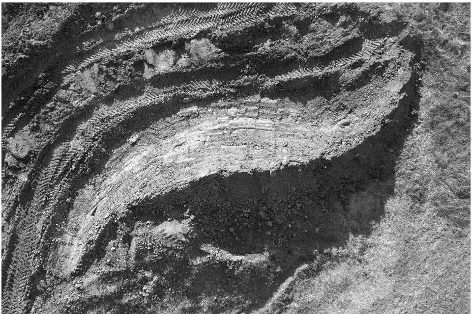
Figure 4.23: Orthophoto of the final geometry of the robotic embankment prototype.
