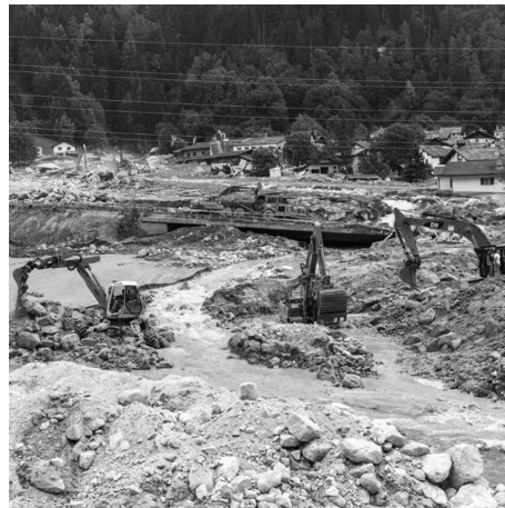
(b) Heavy equipment at work on 23.08.2017.
