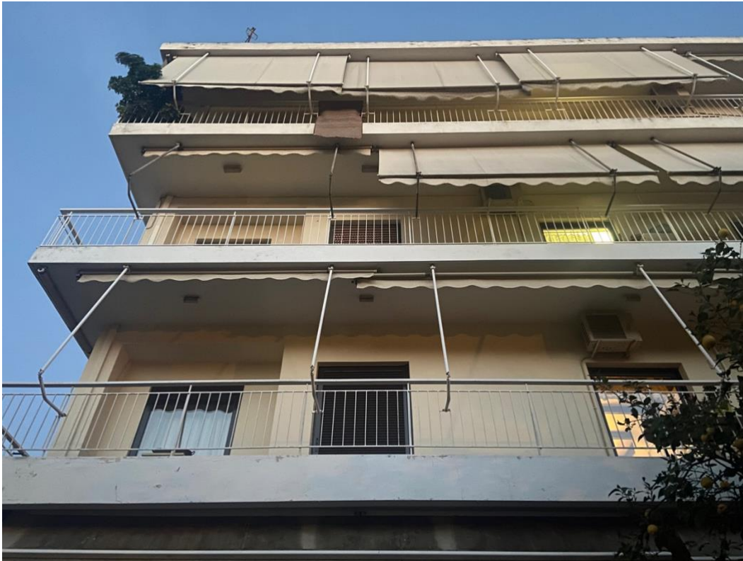
Figure 6. Photograph of a 'polykatoikia' showing the textile awnings in its balconies in Palaio Faliro Athens. Photograph taken by Marianna Charitonidou on 8 April 2020
