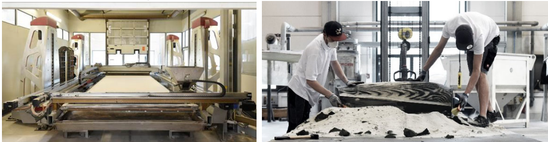
Fig. 6. The binder-jetting 3D printer used for the Smart Slab formwork (left) and the post-processing of one of the 3D-printed formwork parts (right).
