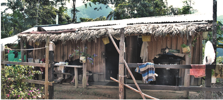
Figure 2: A traditional House in San Francisco. Houses in the region have traditionally been self-constructed using locally available building materials such as rammed earth, bahareque (mud and guadua), and sawn wood. For many, these techniques have several advantages. Foremost, they offer the possibility of repair and upgradations for the residents using the resources at hand. Furthermore, they can easily adapt the spaces that are a part of the local vernacular, and these houses respond better to local weather conditions than structure constructed using concrete blocks and bricks.
