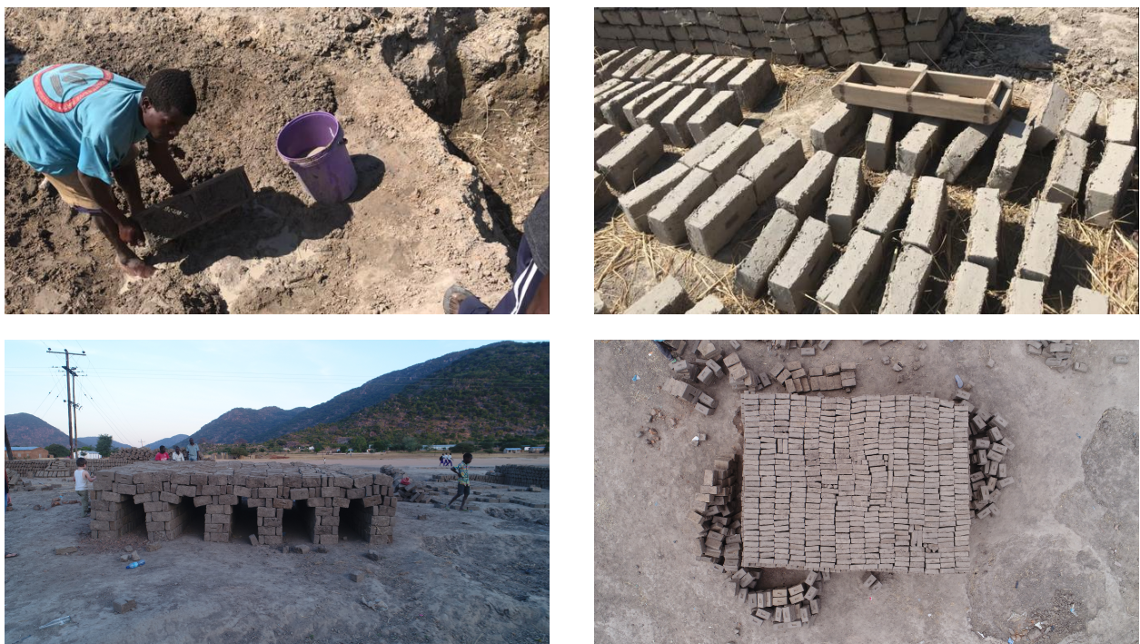
Figure 1.5: Construction of a Scove Clamp out of hand-moulded, dried bricks.
