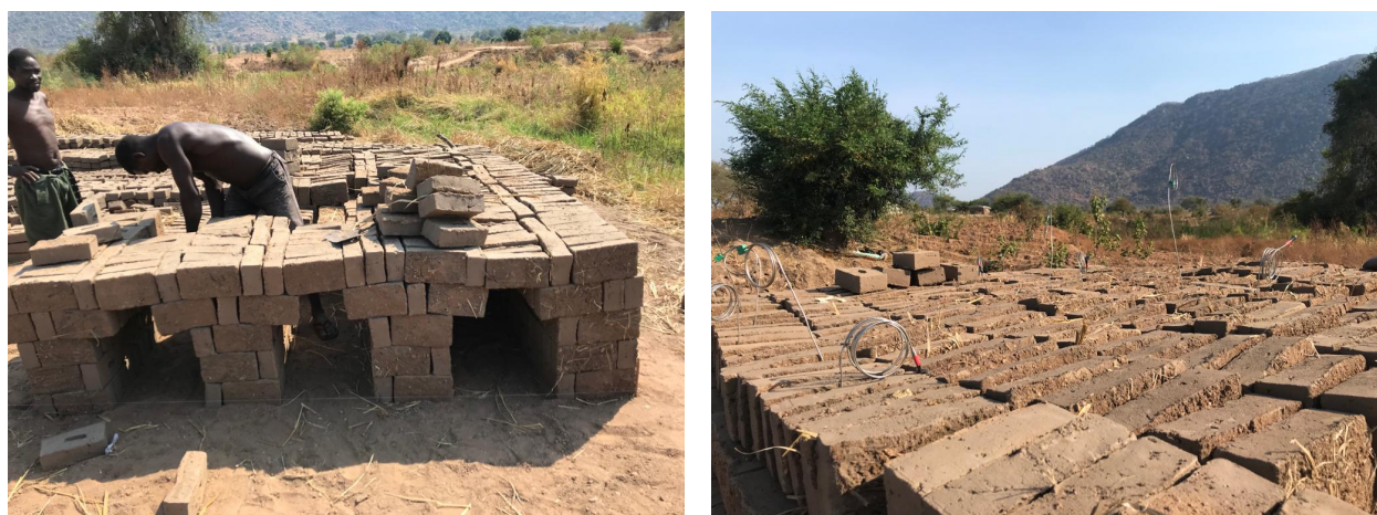
Figure 2.5: Building the oven and installing the temperature sensors.
